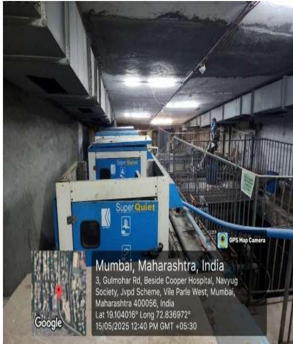
Sewage Treatment Plant
